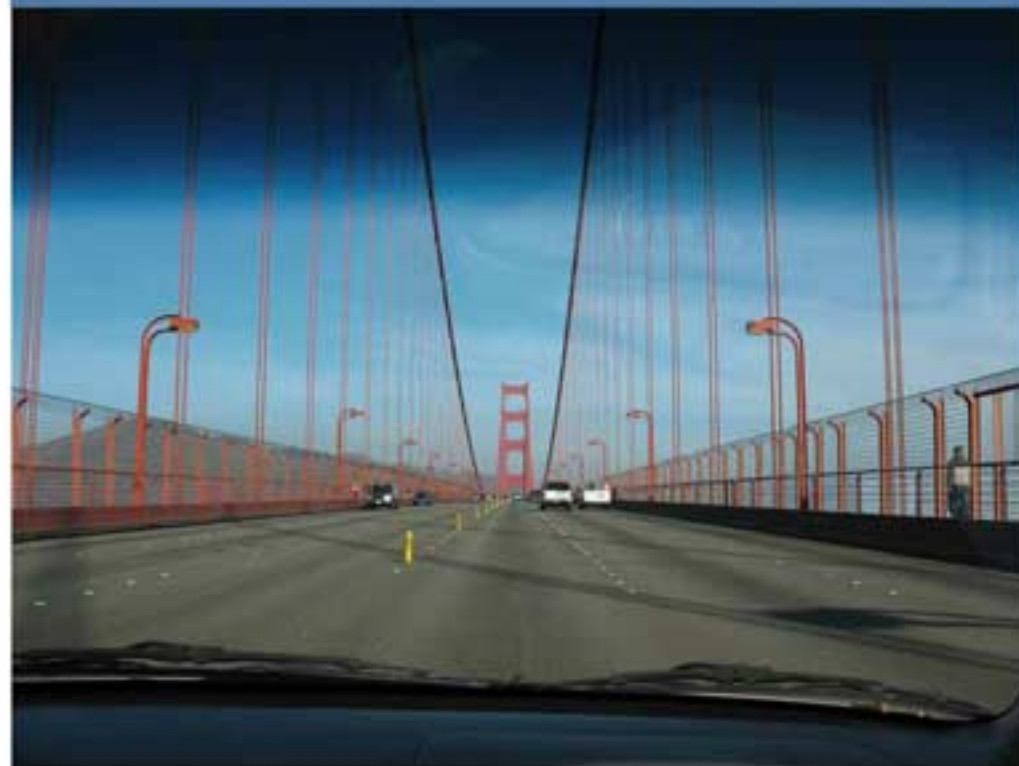
Alternative 2B: Replace handrail with horizontal system - adverse visual impact
